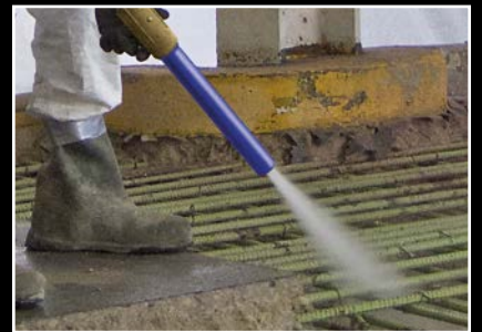
Concrete Repair & Restoration
