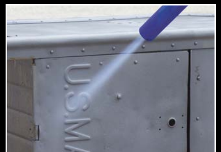
Steel Surface Preparation
